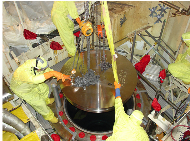
Pump and motor field maintenance activities
